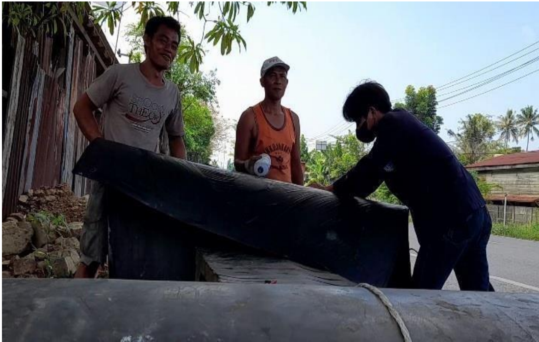
Lampiran 14 Pengolahan Karpet Conveyor
