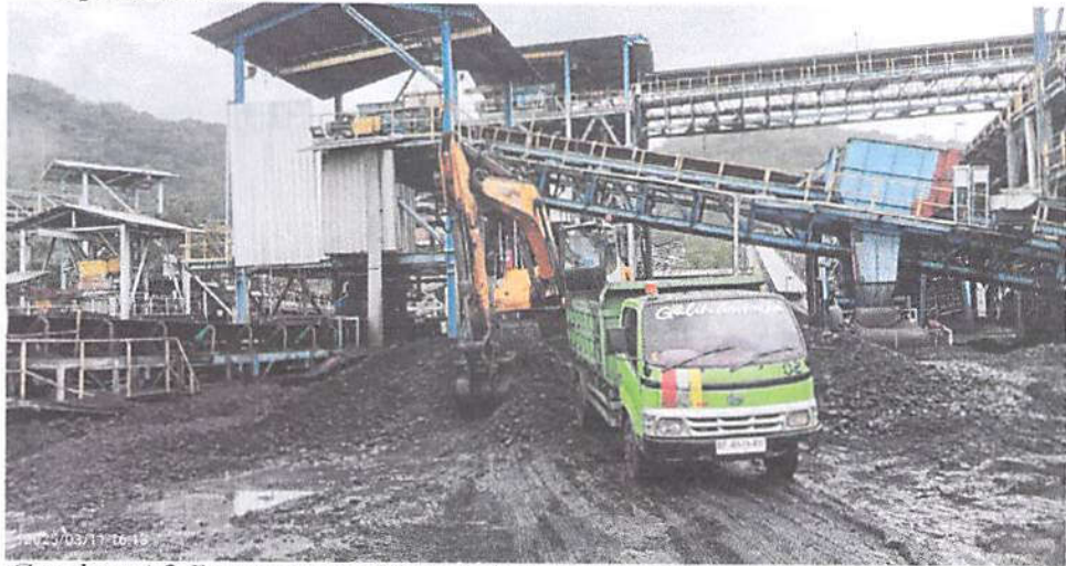
Gambar 4.2 Penanganan Material Oversize di Area Operasional
