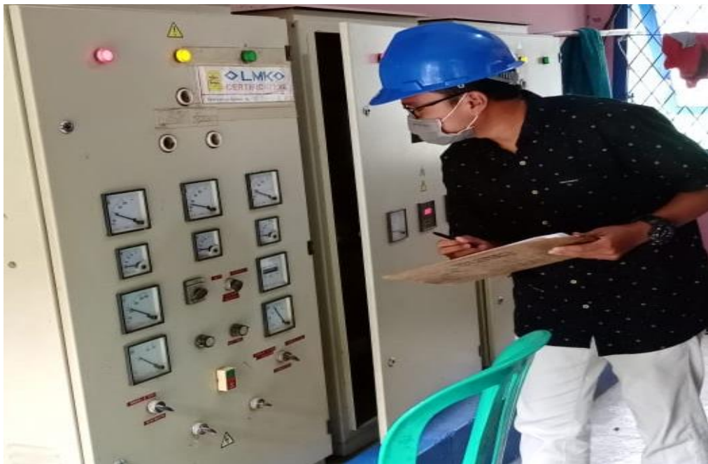
Gambar 2.3.2.4 Pengecekan panel control dan turbin generator
