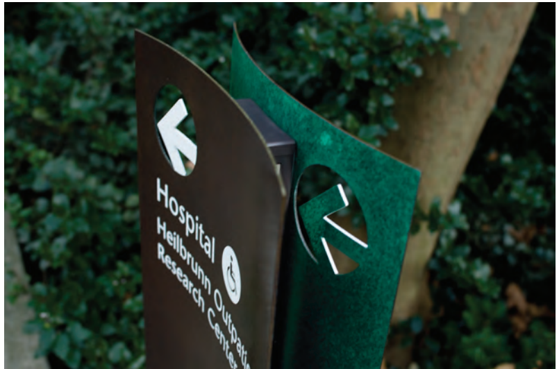
6.65 Metal patina coatings can occur naturally over time or can be applied, as with this chemically accelerated green patina on an oxidized bronze sign at Rockefeller University in New York.
