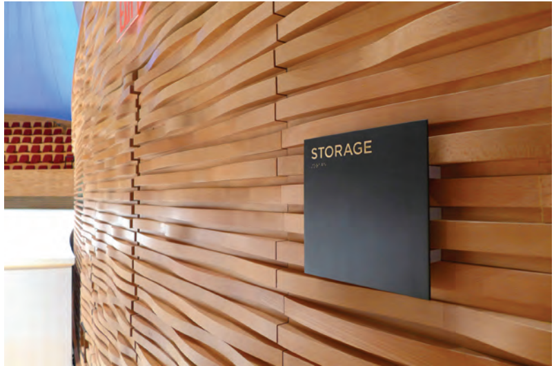
5.74 Identification sign at Stanford University's Bing Concert Hall has cut metal raised characters and raster bead Braille.
