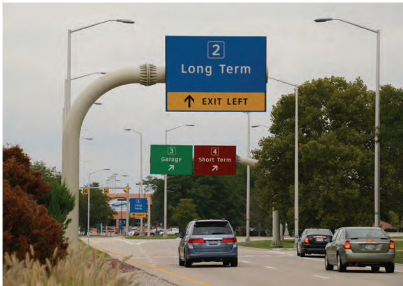
5.39 Different sign panel colors distinguish various destinations to enhance roadway navigation at Dayton International Airport.
