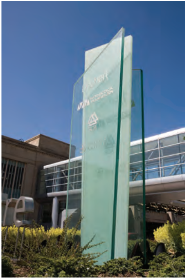
6.43 Three laminated glass panels comprise the tenant identification pylon at Philadelphia's Cira Centre. The middle panel uses a translucent lamination interlayer; the outside panels use an optically clear interlayer.
