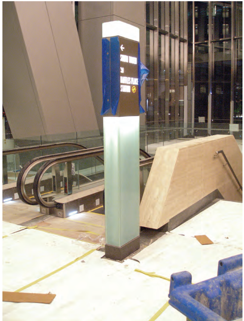
2.40 Observation phase: A finished pylon sign installed onsite still wears some of its blue protective sheathing.
