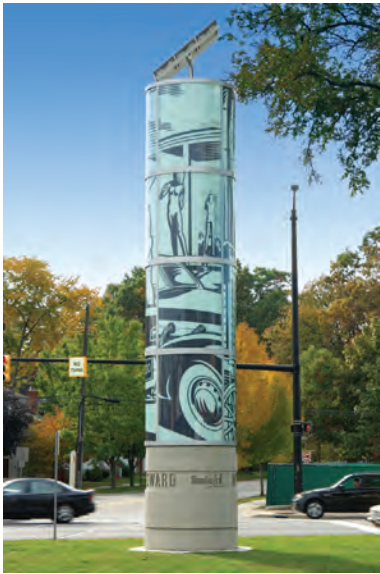
6.44 Curved glass panels are laminated with a printed translucent interlayer for the Woodward Avenue Tribute towers in Detroit. Interlayers can be printed in full color or black and white.
