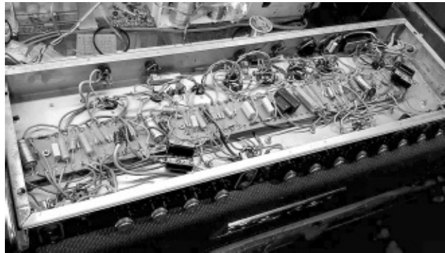
Figure 23.43: Point to point wiring is labor intensive and potentially prone to assembly errors. Photo courtesy of Amplifier Experts.
