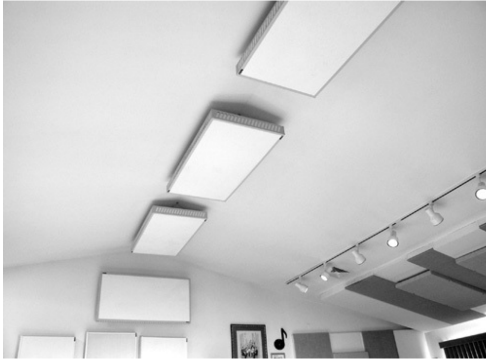
Figure 20.4: The ceiling in Ethan’s home studio is peaked, rising from 8 feet high at the front and rear walls to 12 feet in the center. Absorbers hanging a few inches under the peak reduce the focusing effect that occurs with concave surfaces.
