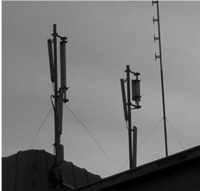
Figure 20.10 Mechanical downtilt of base station antennas. The downtilt can also be handled electrically which provides possibility to tune the angle remotely.
