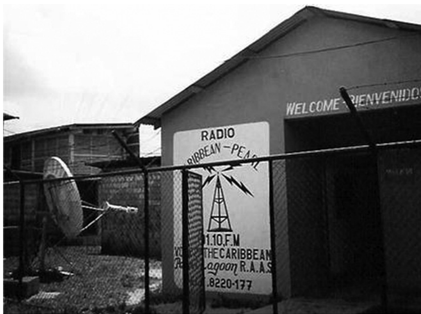
Figure 16.12 An example of VSAT station in Nicaragua, Laguna de Perlas, which is isolated from other cities as there are no car routes, only a river leading to the village. The parabolic antenna located outside, and the actual VSAT equipment with respective computer located indoors can be used to connect to Internet with over 100 kb/s data rate. Photo: Jyrki T.J. Penttinen.
