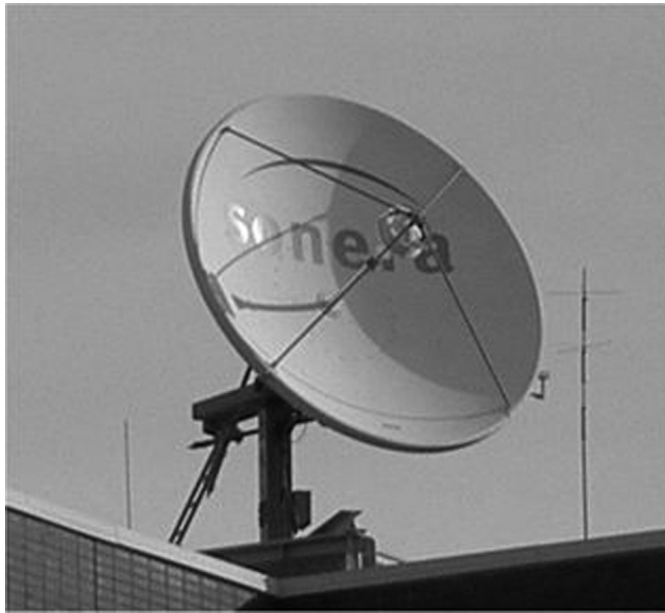
Figure 16.5 An example of parabolic satellite antenna that is fed via the head located at the front of the antenna.
