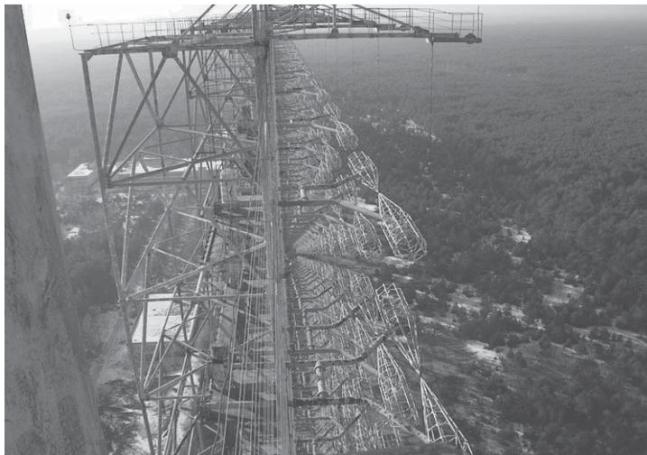
**Figure 1.3.** Russian Woodpecker OTHR radar. Photograph obtained via the Internet (<http://passingstrangeness.wordpress.com/2010/04/23/the-russian-woodpecker/>).
