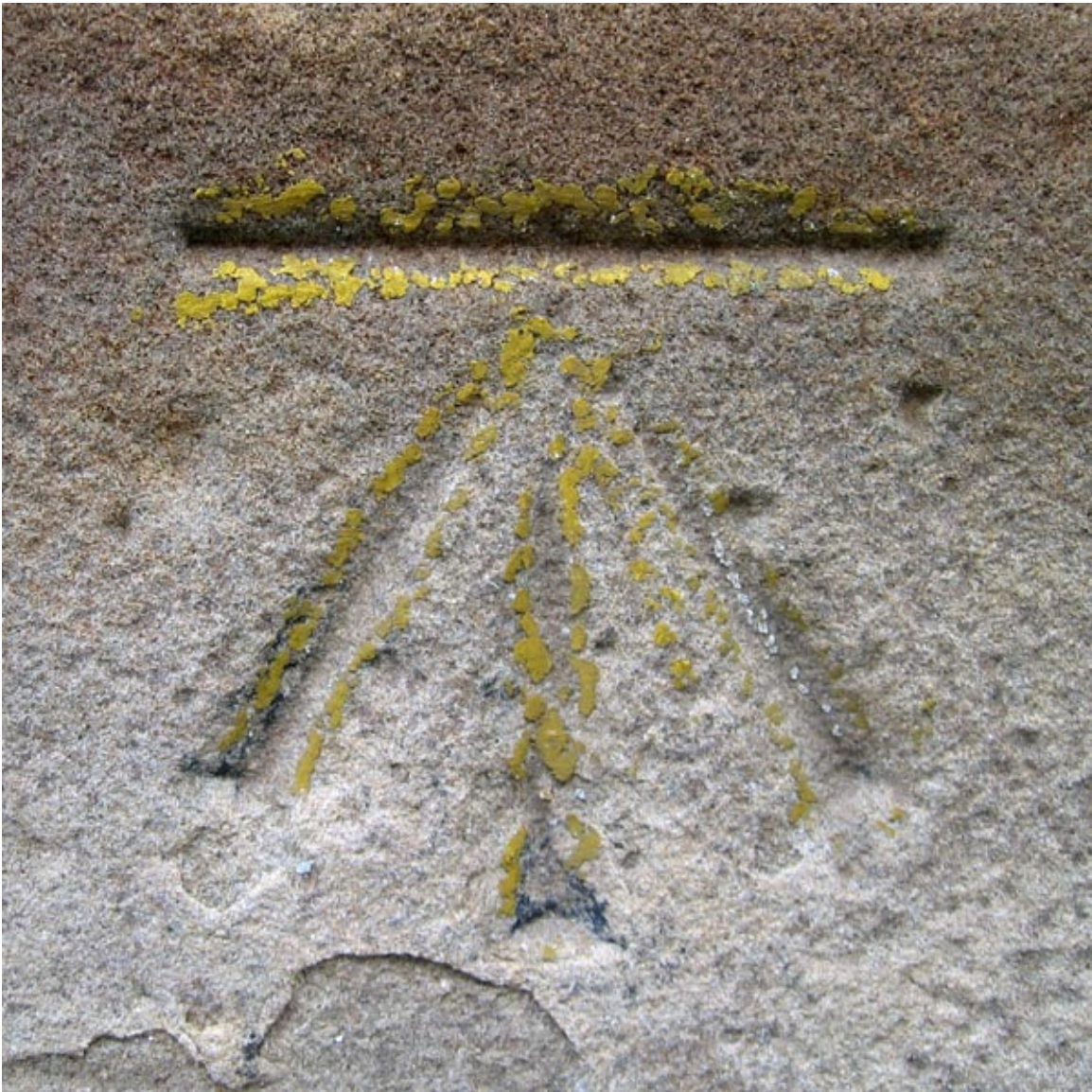
Figure 5-4. An Ordnance Survey cut mark in the United Kingdom. “BmEd” licensed under Creative Commons.
