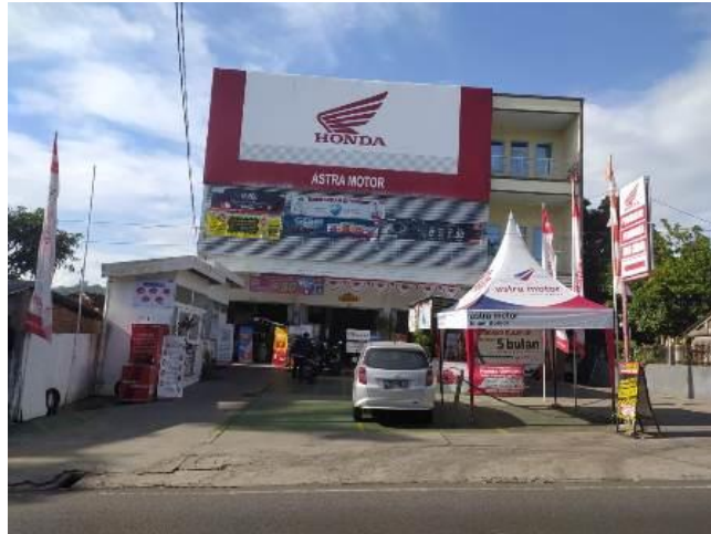
Gambar 3.5 . Gedung PT. Astra International tbk – HSO Lampung III
